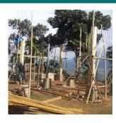
The main structure is elevated, allowing better airflow around the building due to its exposure to the elements and site position. In turn, this will help with cooling during summer and ensure the kids are out of harm's way from the downpours during the rainy season.
